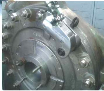
◀ PSD-3 Bolt tightening of Centrifugal pump casing
